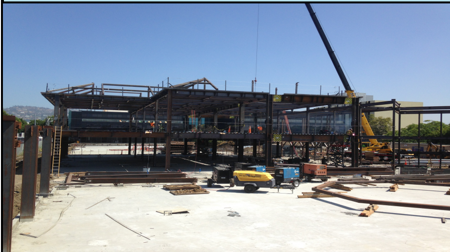
North structure of Section B from Charleville. Roof structure visible near Robetson Blvd.
