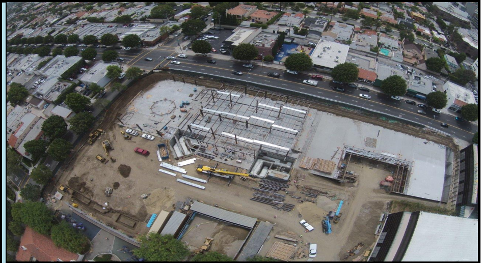
Aerial view of site showing steel erection and structural footings at slab on grade.
