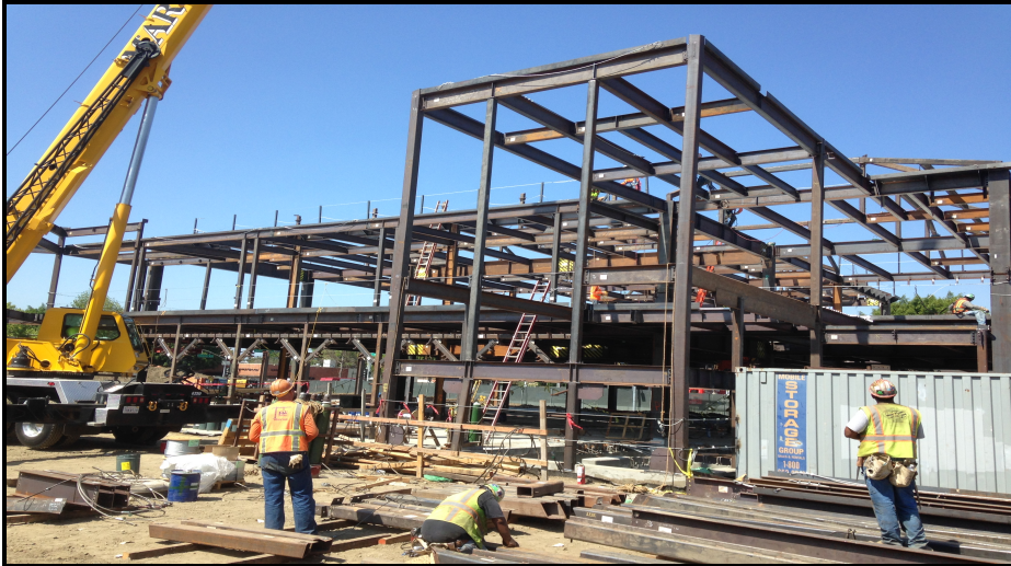
Structure for the elevator tower north east side. North section nearly complete.
