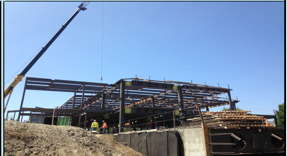
North end of structure from parking ramp.
