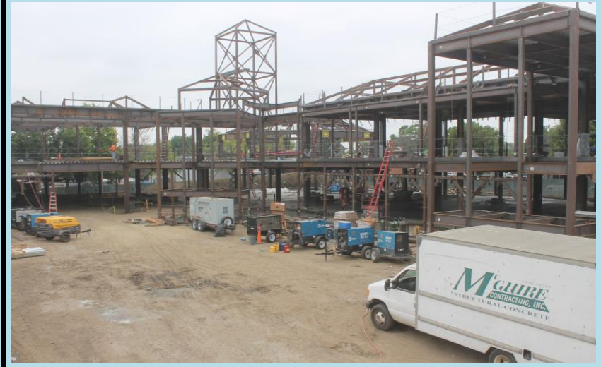
Image from workzone time lapse camera
