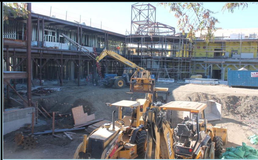
Image From Workzone Time Lapse Camera
