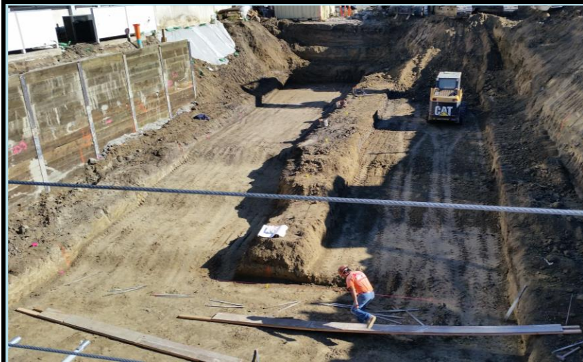
Parking Garage Ramp
