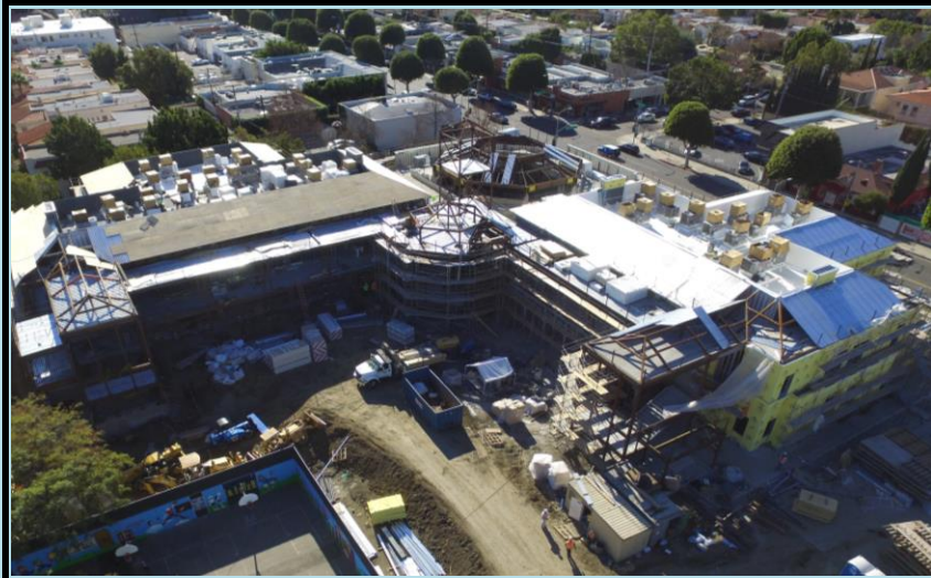
Building B Aerial
