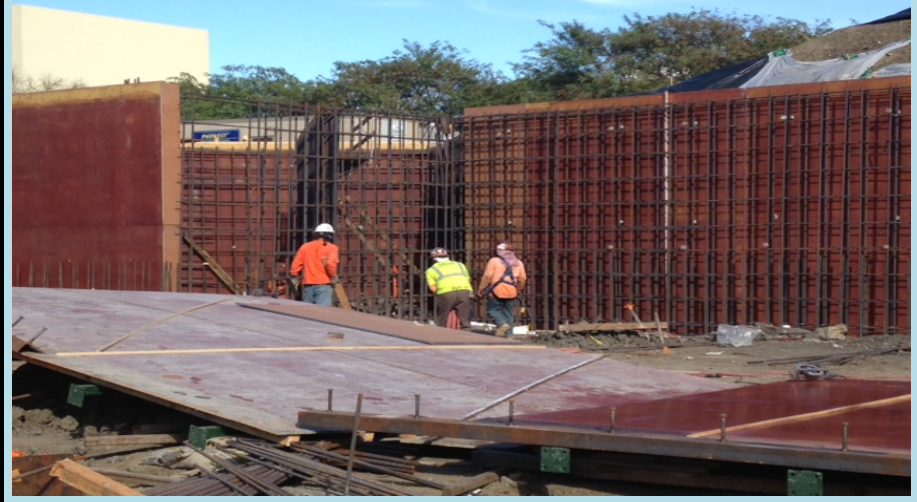
Rebar for retaining wall
