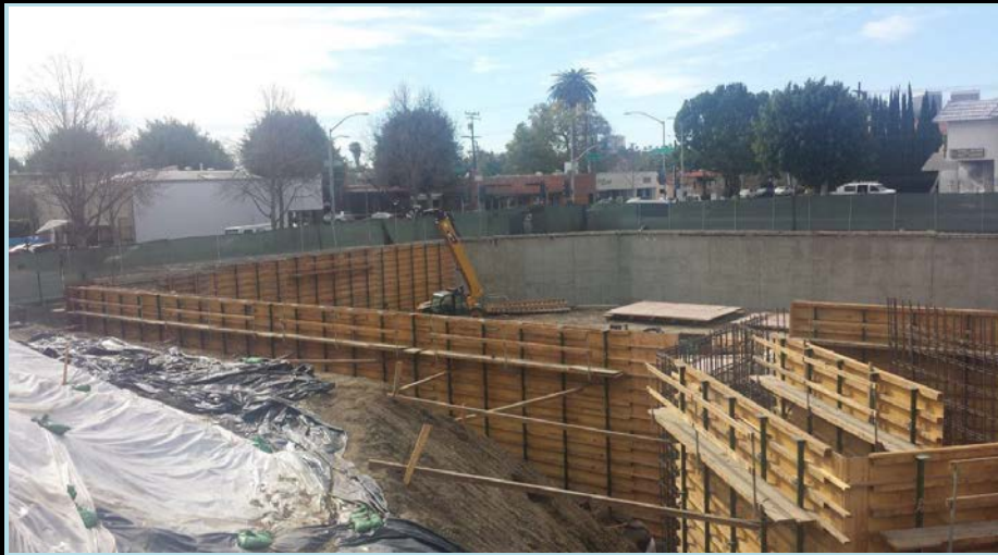
Progress with basement retaining wall
