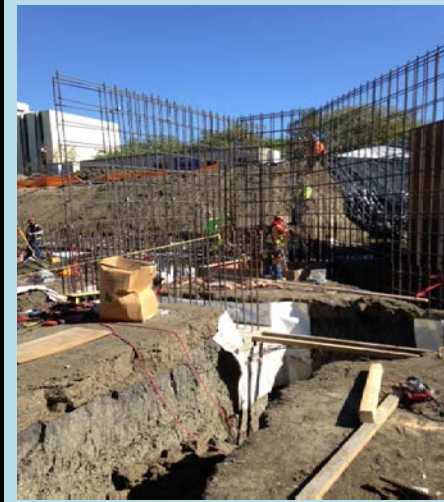
Progress with footings and retaining wall
