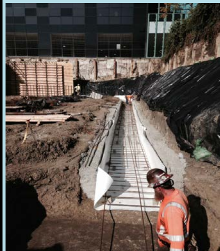
Footing work. Note the grey "slurry" poured behind the waterproof membrane to mitigate the rain damage
