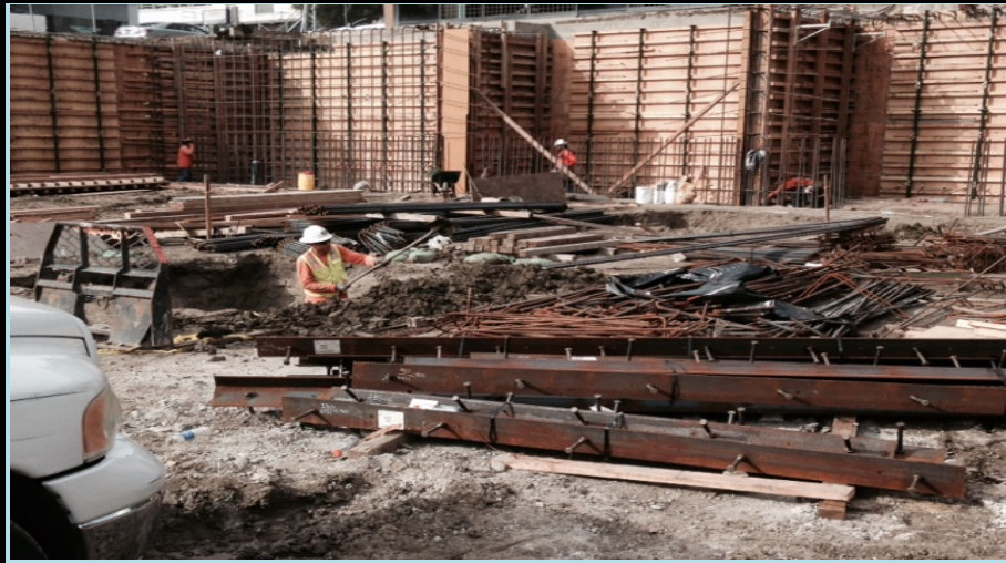
Basement formwork and steel
