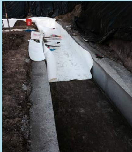
Footing work. Note the grey "slurry" poured behind the waterproof membrane to mitigate the rain damage
