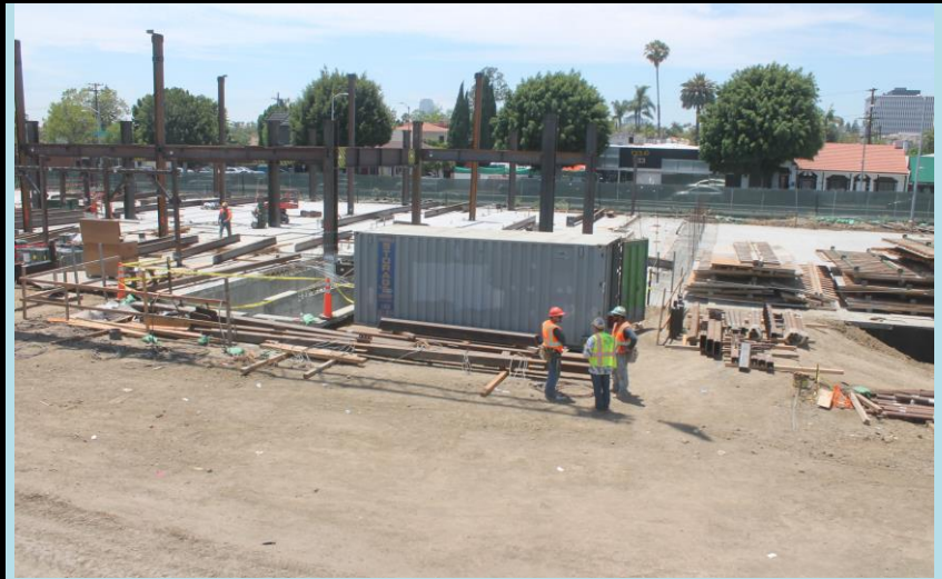
Image from workzone time-lapse camera.
