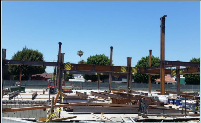
First Floor Steel Erection Ongoing.
