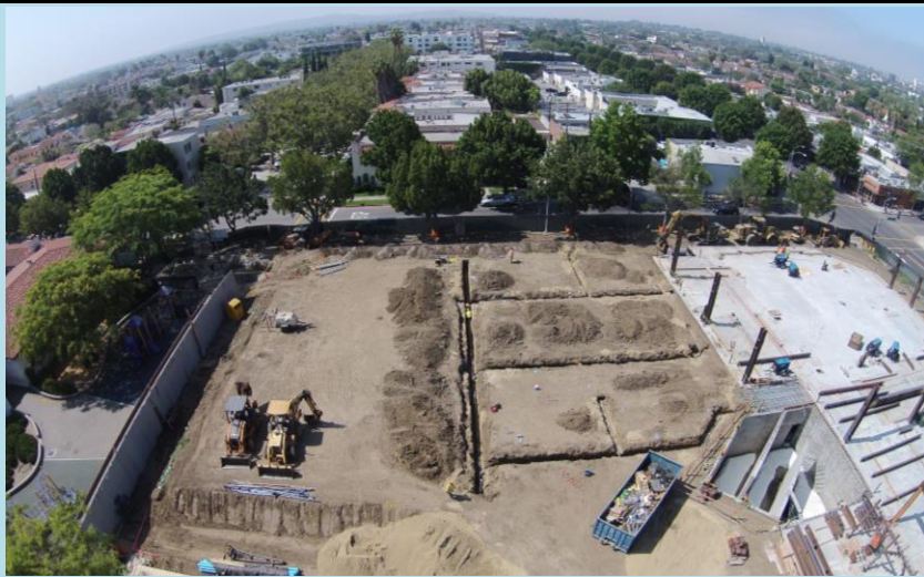
Area "A" underground plumbing. Formerly known as "Husky Hill".
