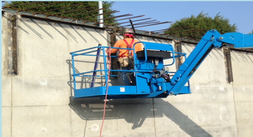
Preparing concrete wall for steel
