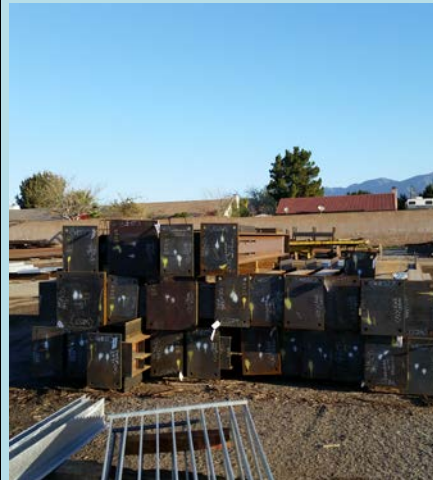
Steel fabrication at the steel yard
