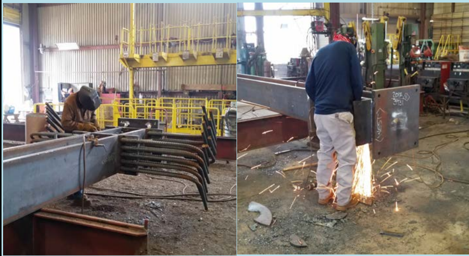
Steel fabrication at the steel shop. Note the size of the rebar. IOR has visited steel shop.
