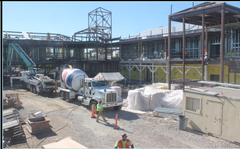
Image From Workzone Time Lapse Camera
