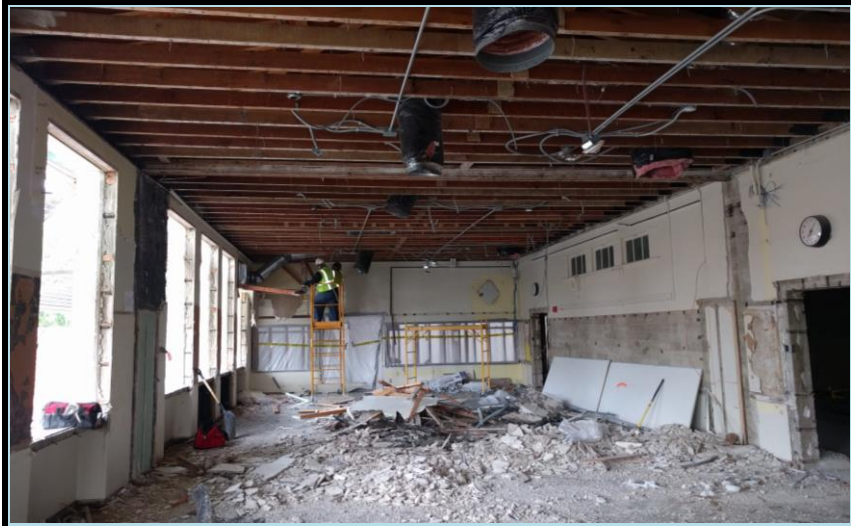
Bldg A 2nd Fl Demo
