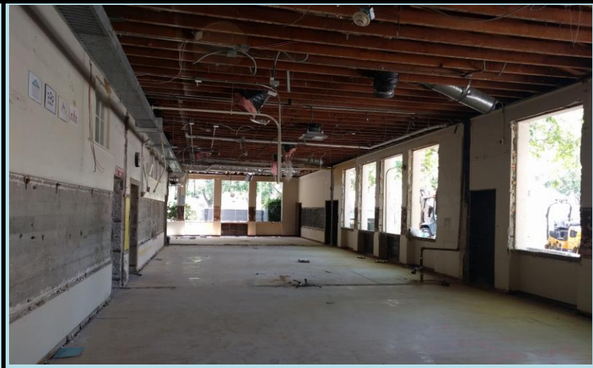
Bldg A 1st fl Demo
