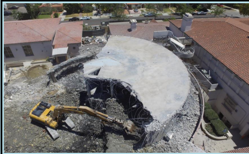
Building E Demo
