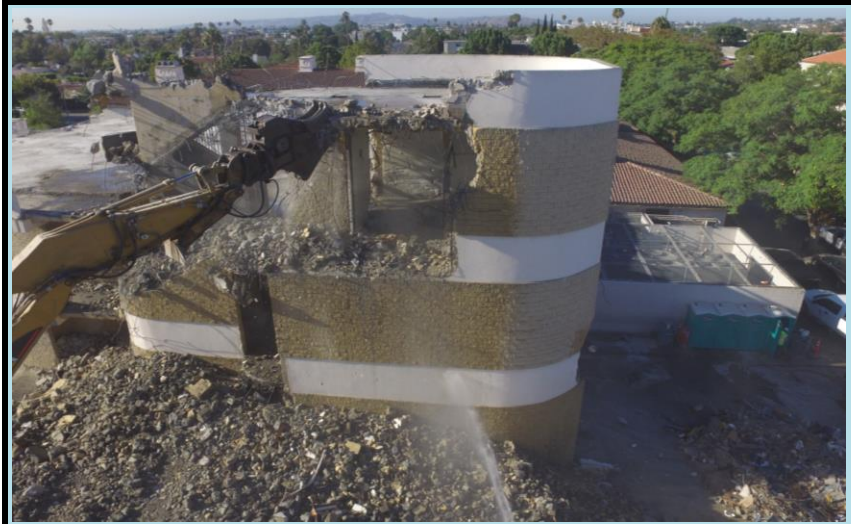
Building E Demo
