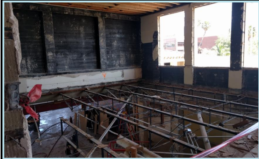
Bldg. A 2nd floor demo
