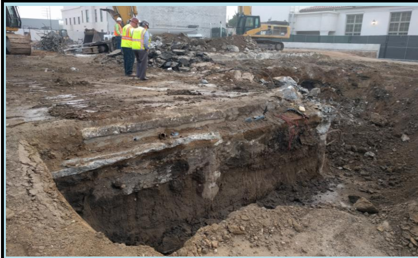
Bldg. E Footing Demo
