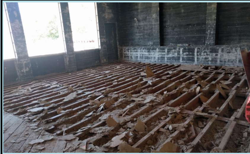
Bldg. A 2nd floor demo
