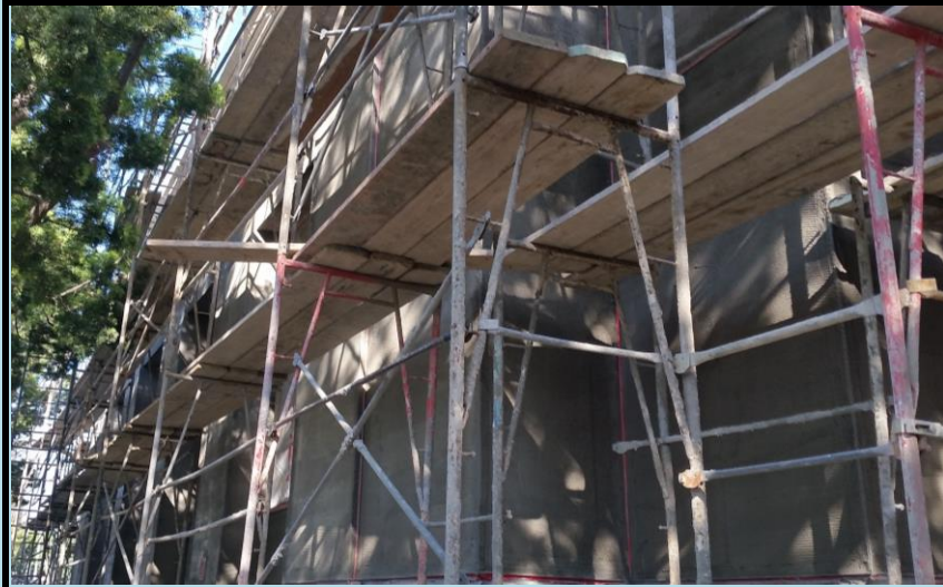
Plaster at Charville BLVD
